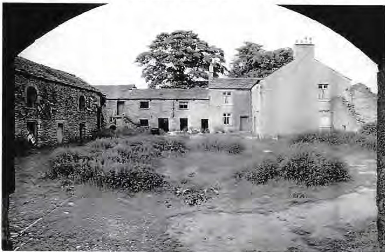
Birchencliffe Farm Yard before rebuilding
