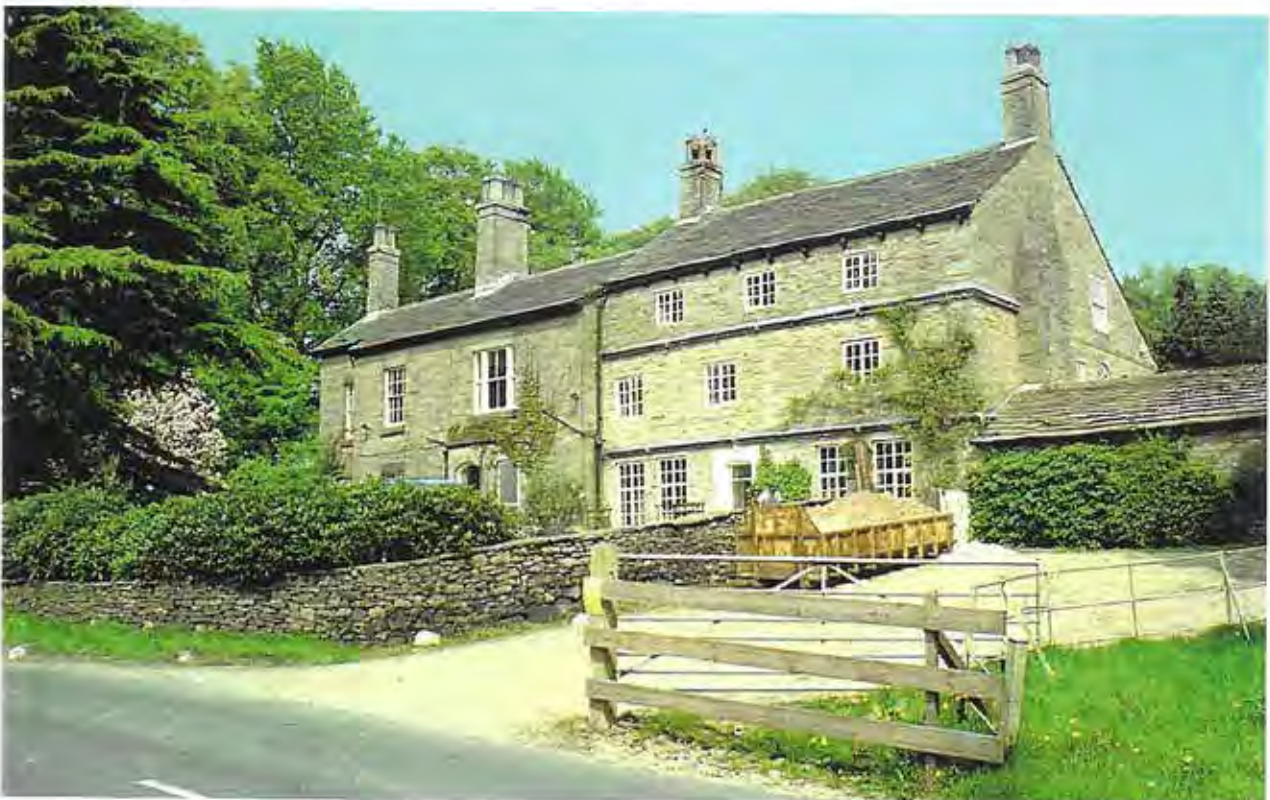
Pott Hall, May 2000, as conversion to apartments commences
