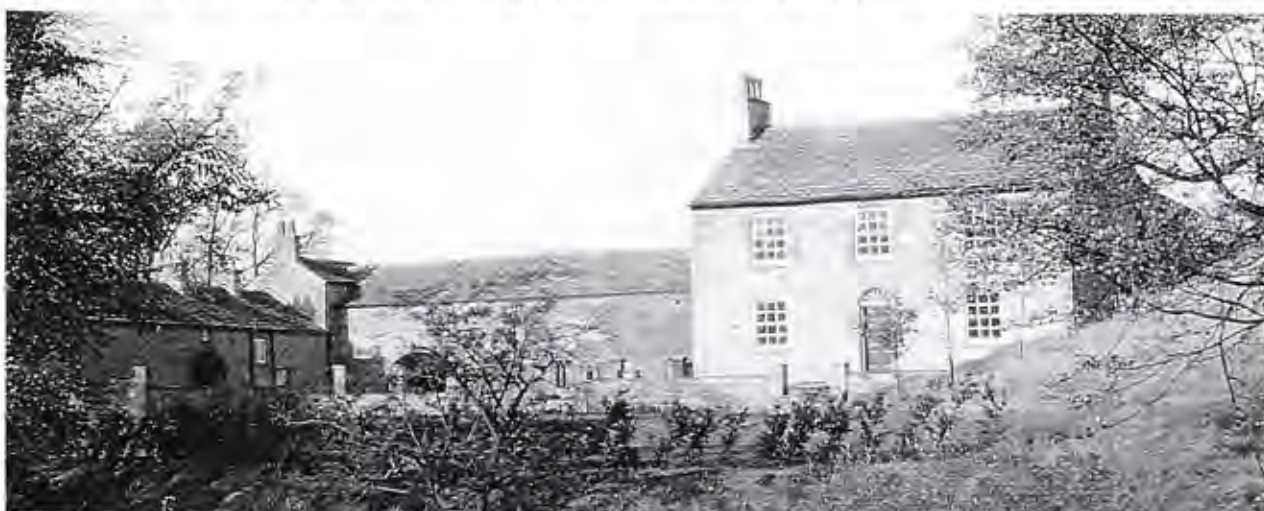
Birchenccliffe Farmhouse after rebuilding
